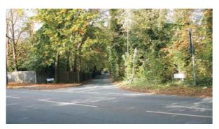
Advance signing will be improved at the junction of The Common and Warren Lane. This will involve moving the change of speed limit further into Warren Lane by about 60 metres, which should eliminate sign clutter and reduce vehicle approach speeds.
